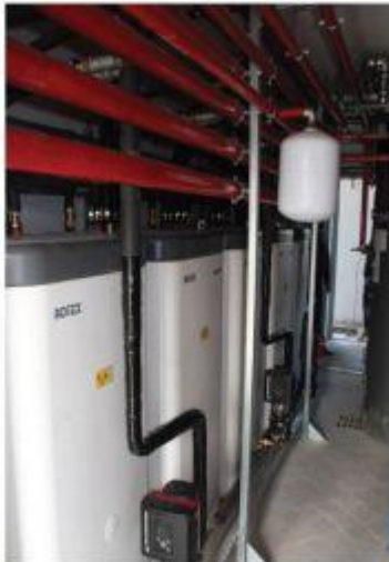
Centrale termica: serbatoi di accumulo acqua calda 500lt. Mechanical room: hot water storage tanks of 500 litre capacity.
